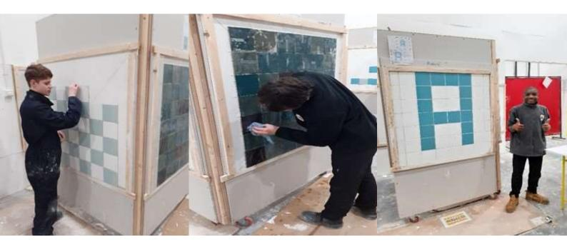
In the above photos, the Nurture groups 5 & 6 have been learning how to tile and are now working on their assessment pieces. This has involved them working out a design on paper then transferring it onto the board. They have had to set out their battens plumb, then locate the centre of the boards and tile out from the centre line. They have also had to learn how to cut tiles to size and have shown fabulous skill across all of these elements.
